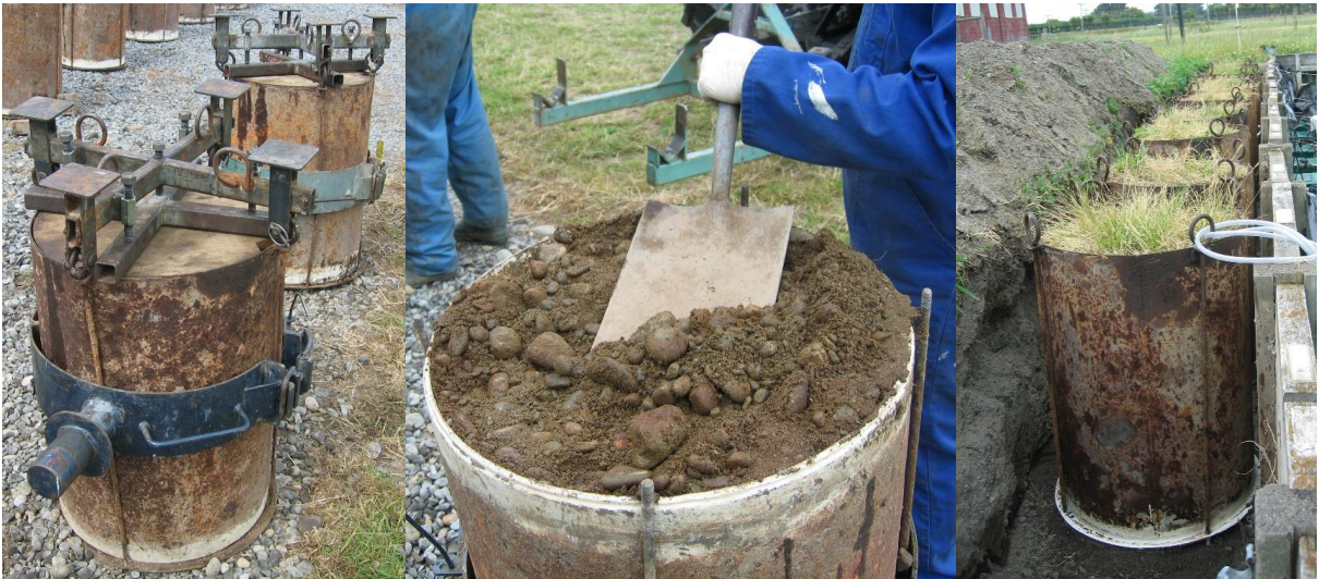
Figure B. 2. Left – Right : Lifting frame attached with the lysimeters to invert upside down; preparation to install drainage system; placed in the trench, before the surrounding filled with soil.
