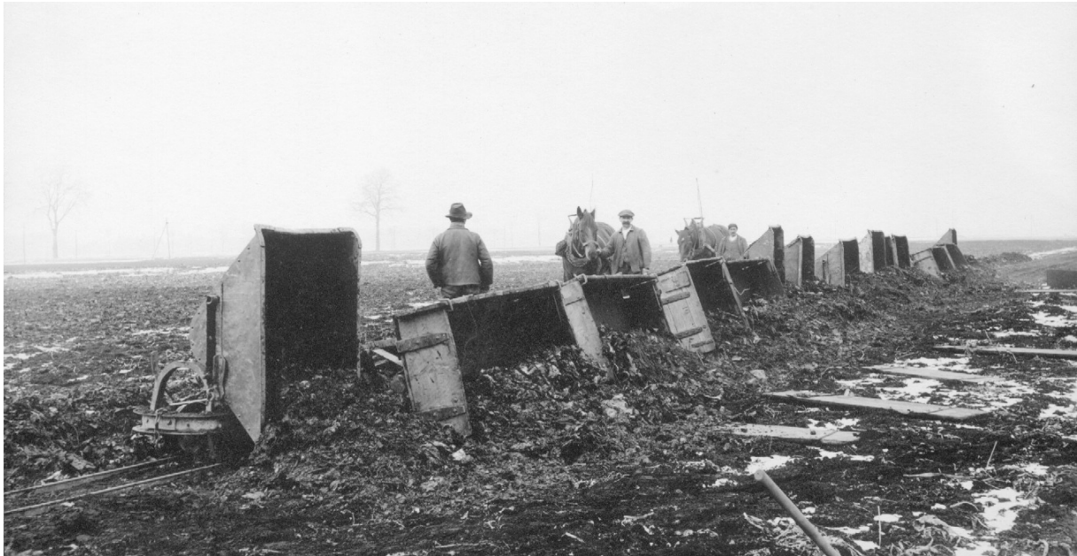
Figure 2-4: Waste transport in tipping lorries and disposal on the field. Origin of photo: Archives of the Witzwil prison.
