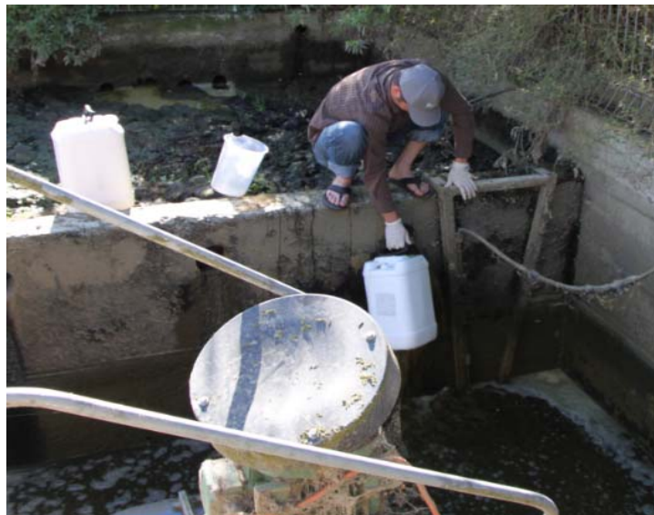
Plate 10– Image of effluent pit and collection of effluent for slurry application. (Photograph by M. Simmler, personal communication, 2011)
