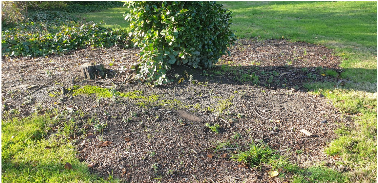
Figure 3.11. Photograph of an area of interest for targeted sampling in the RZ off Harvey Terrace, Richmond. Note. This area is an example of an area that can be targeted for sampling as it has a higher likelihood of having elevated soil HM concentrations (bare patch of soil that is next to vegetation and has visible brick fragments).
